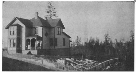
[1521] J.F. Pike Residence, 1621 1st Avenue North, March 1891.
